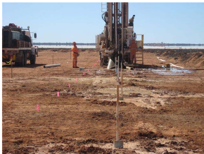
Figure 2: Drill rig drilling water barrier lines
