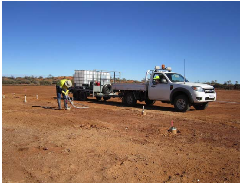
Figure 3: Applying the geopolimer to the drill holes
